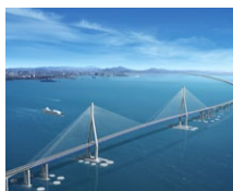
Incheon Bridge (KR)
